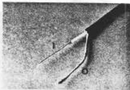
4. Trim insulation an inch from splice point, twist sheath (O) and remove 1/4 in. of insulation from end of inner wire (I).
